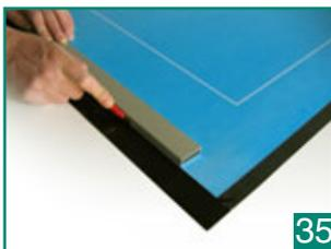
After mounting cut away the unnecessary strips.
